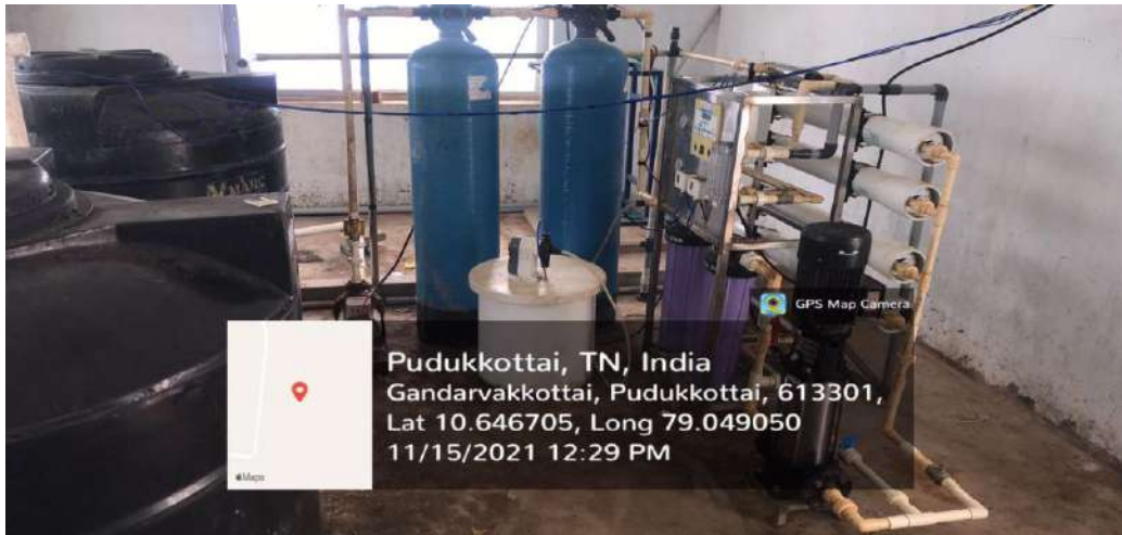
Reverse Osmosis Plant (RO)
