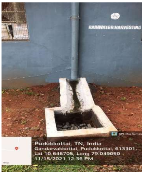
Rainwater Harvesting system at Block IV
