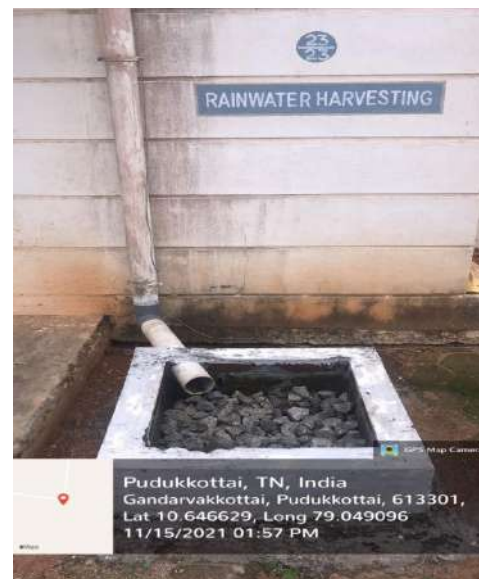
Rainwater Harvesting system at Library
